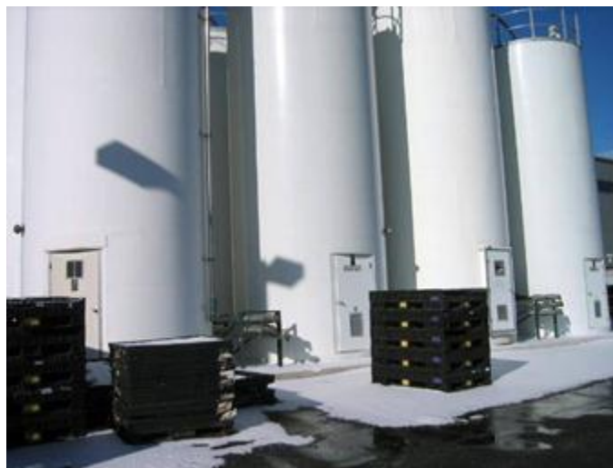
Example of a confined space – storage silo.
